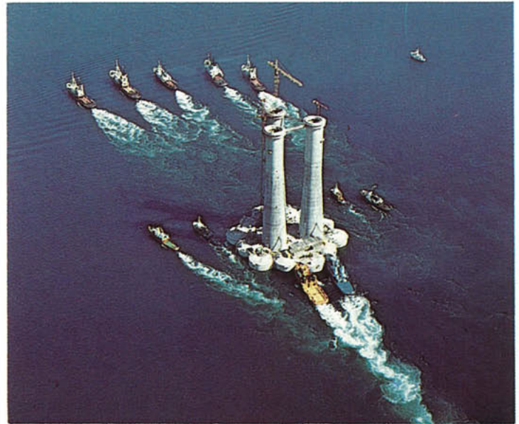
2) August 1976: The concrete gravity base structure of the Statfjord A platform was towed from Stavanger to Stord.
