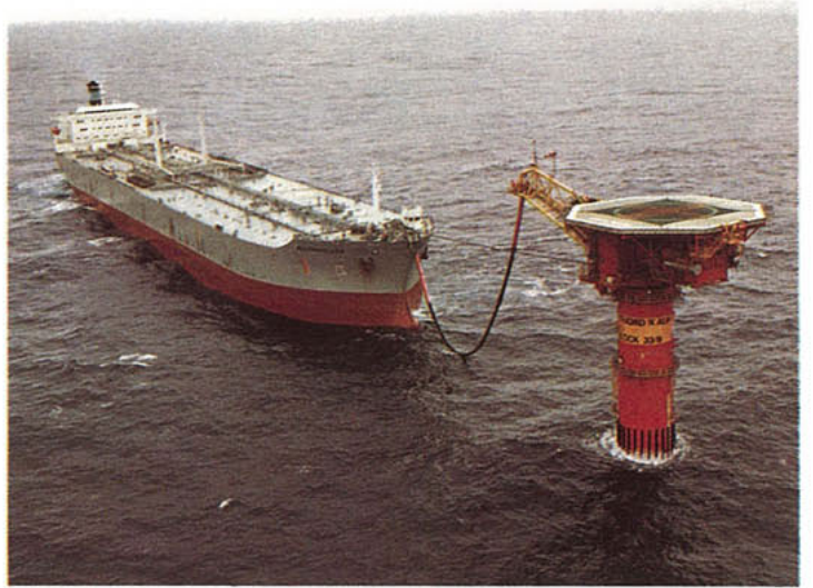
8) December 1979: The first oil from the single point mooring buoy on the Statfjord field is loaded into Polytraveller .
