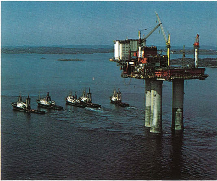
4) May 1977: The platform was towed out to the field under good conditions.
