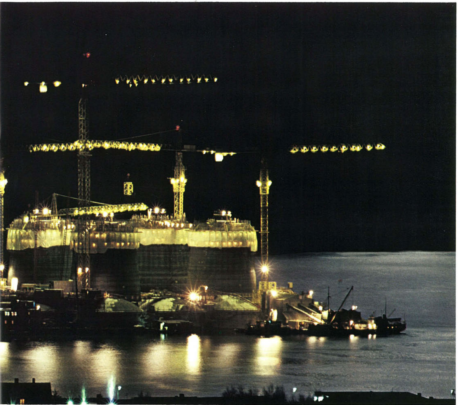
Above: The concrete gravity base structure of the Statfjord B is being cast in Stavanger by Norwegian Contractors. Below, this page: Modules are lifted into the steel deck frame of the Statfjord B, under construction at Moss Rosenberg Verft in Stavanger. Below, opposite page: Pipeline welding for Statfjord B.
