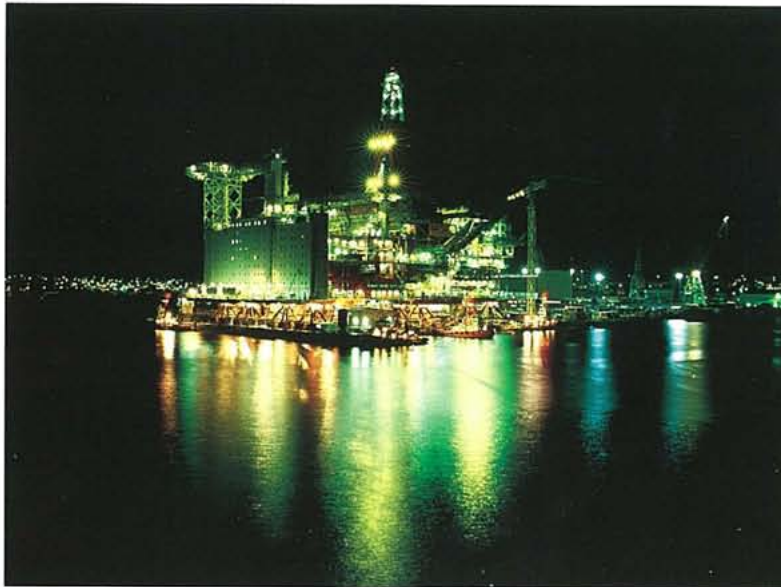
The Statfjord C deck was mated with the concrete base structure in Yrkjefjorden north of Stavanger in February 1984. Above we see the steel deck at Moss Rosenberg Verft in Stavanger before tow-out to Yrkjefjorden.
