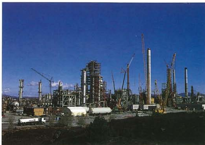
The construction site at Mongstad.
