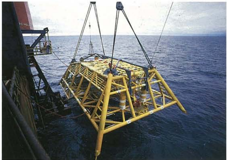
The Tommeliten template lowered to its seabed site.
