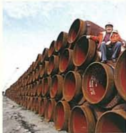
A thousand kilometres of pipe for Zeepipe. Each of the 12-metre pipes weighs up to 25 tonnes.
