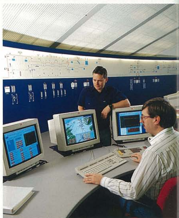
A substantial share of Norway's gas deliveries to the Continent is handled from the control room at Bygnes north of Stavanger.
