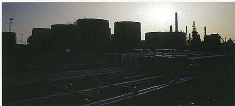
The Mongstad refinery.
