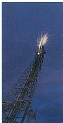
Extinguishing the flares on Gullfaks A and C reduces the emission of greenhouse gases.
