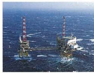
The 16/11 area in the Norwegian North Sea has become one of the most important hubs for Norway's gas transport systems. Six pipelines now run through the 16/11-E riser platform, which was commissioned in 1994.
