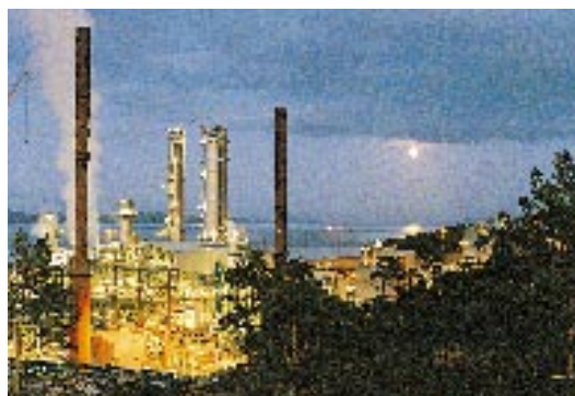
THE METHANOL PLANT AT TJELDBERGODDEN WAS OFFICIALLY OPENED IN JUNE 1997.
