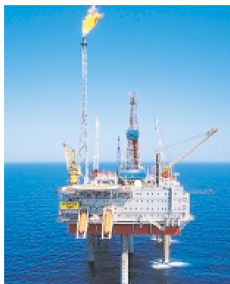
DENMARK'S SIRI FIELD CAME ON STREAM IN 1999.
