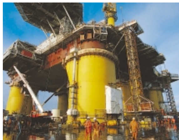
OUTFITTING ÅSGARD B IN STAVANGER.
