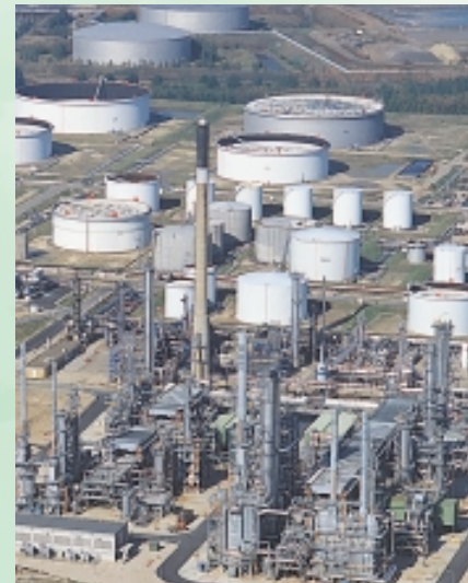
STATOIL'S REFINERY AT KALUNDBORG IN DENMARK.
