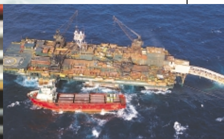
LAYING EUROPIPE II.
