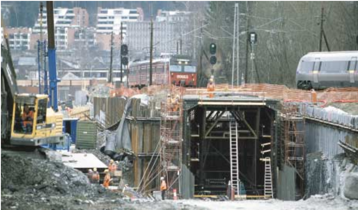
Construction works at Jong. (Photo: Rune Fossum)
