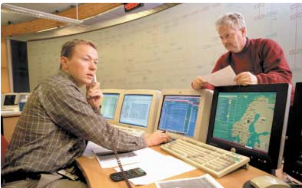
The Statnett Control Center represents the core of the daily coordination and control of the Norwegian Power System. A continuous coordination and monitoring of electricity "highways" is carried out on a 24hrs basis. Kristoffer Sletten (left) and Kjell Sand are seen in the midst of coordination procedures.
