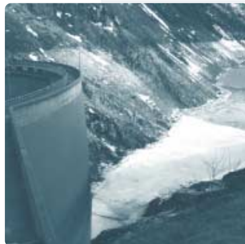
Nearly drained, this Norwegian hydro electric power reservoir, Zakariasdammen in the Roldalsvassdraget showed a cubic content of only 11 million m 3 in April, 2003. Maximum capacity is 70 million m 3 . The reservoir is located in the Møre area and belongs to Tafjord Kraft.
