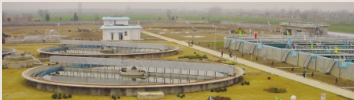
GOOD REFERENCE: The order for this municipal purification plant in Suzhou in China was secured by GIEK guarantees.
