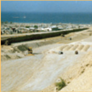
Construction site in Assaluyeh in Iran. (Picture: Statoil)
