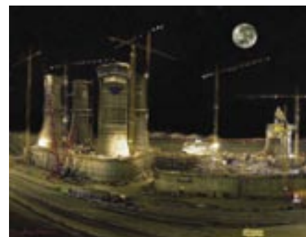
Aker Kvaerner has revitalised Norwegian concrete technology to construct two concrete gravity-base structures in Sakhalin (Photo: Aker Kvaerner).
