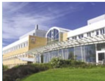
NILU's Head Office is located just north of Oslo.
