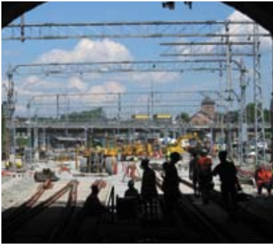
Construction work at Asker station, summer 2005. Photo: Olaf Bjerknæs
