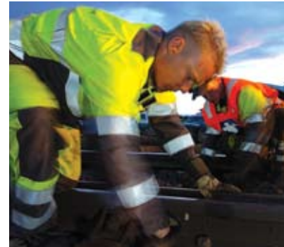
Track maintenance technician Arild Kvaal works on a track switch, while Vegard Lade acts as lookout. Photo: Øystein Grue
