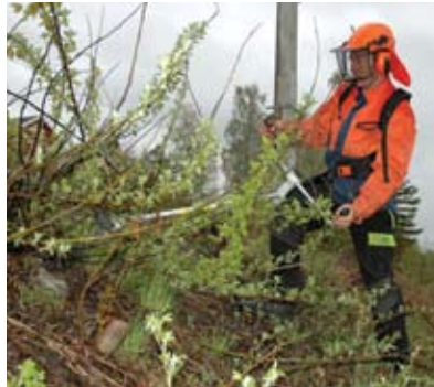
Clearing vegetation at Bleiken station on the Gjøvik line. Photo: Njål Svingheim
