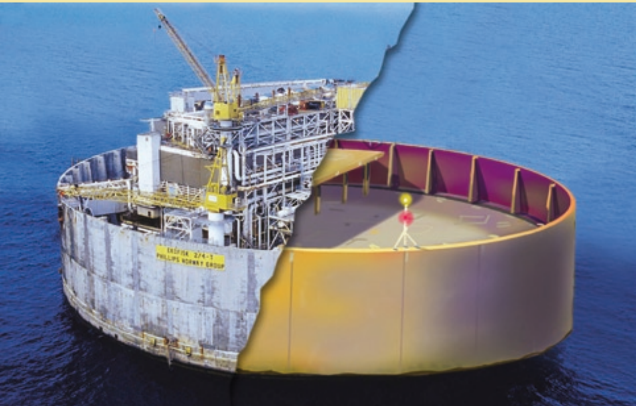
Figure 6.2 Illustration of the Ekofisk Tank before and after removal of the topsides
