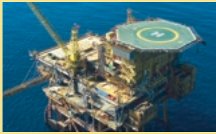
Figure 6.1 Drilling and production installation DP2, to be removed from the Frigg field
