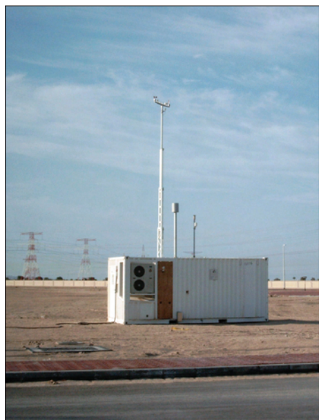
Air quality measurement station in United Arab Emirates.
