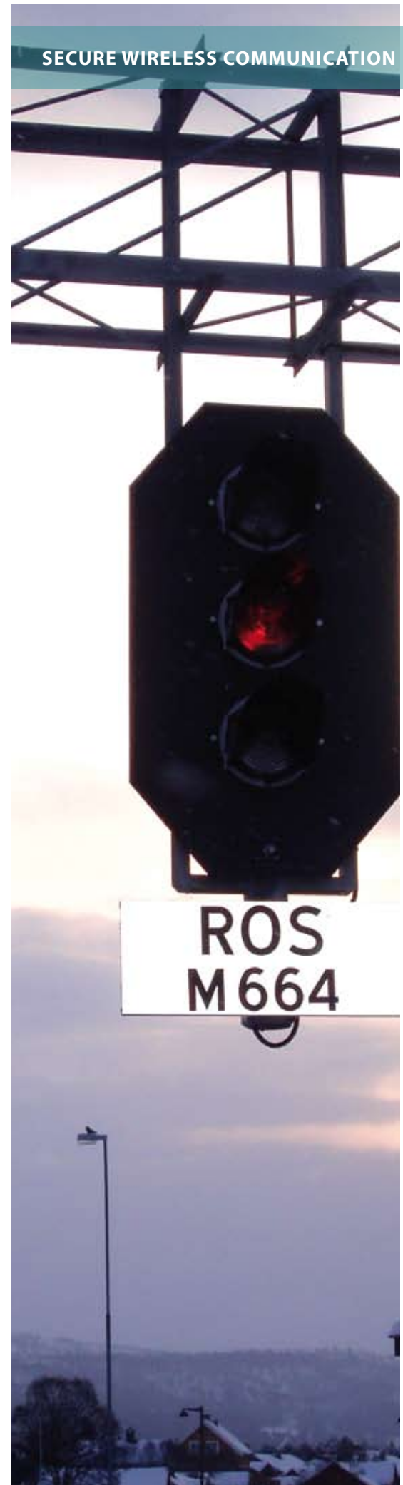
Colour-light signal with location code: 4 400 colour-light signals on the network will be dispensed with when ERTMS takes over.
