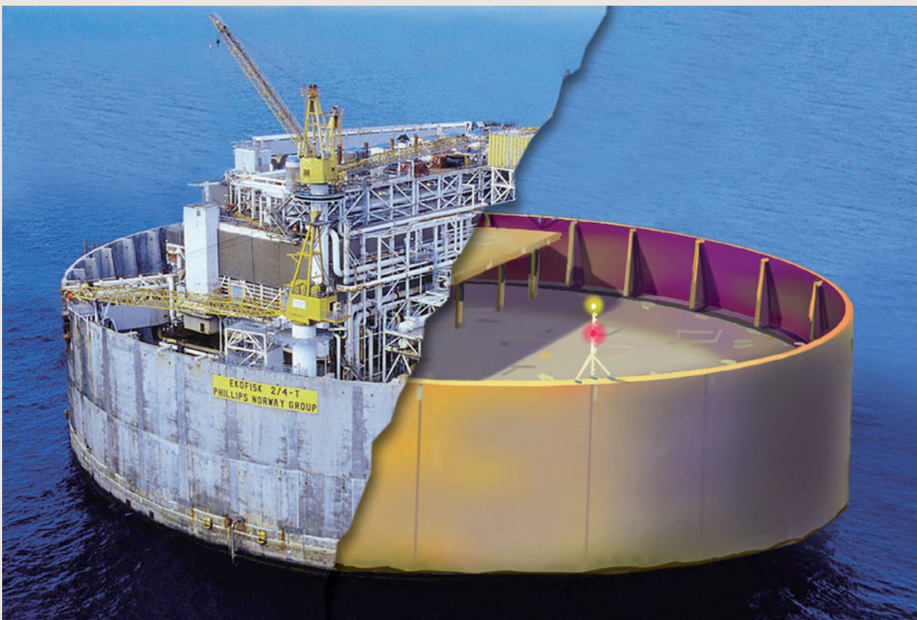
Figure 7.2 Illustration of the Ekofisk Tank before and after removal of the topsides
