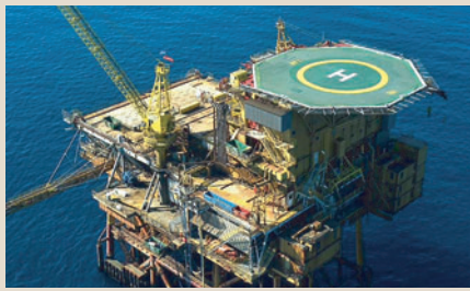
Figure 7.1 Drilling and production installation DP2, to be removed from the Frigg field (Source: Total E&P Norge AS)
