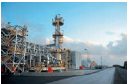
Kollsnes. At Kollsnes gas comes ashore for further processing before it is transported in pipelines to customers in Europe
