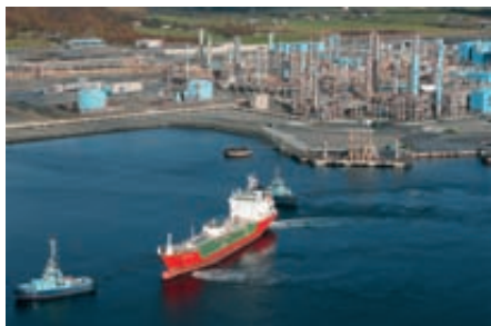
Kårstø. Kårstø is currently preparing for the future with the KEP2010
