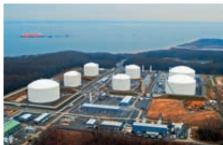
Cove Point. Cove Point with the additional capacity almost finalised and Arctic Princess discharging at the pier.
