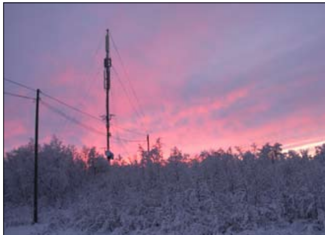
This means that the same extensive, integrated TV services provided by NRK are available to everyone throughout the country. Beautiful winter atmosphere at the transmitter near Kautokeino. Photo: Jon-Annar Fordal
