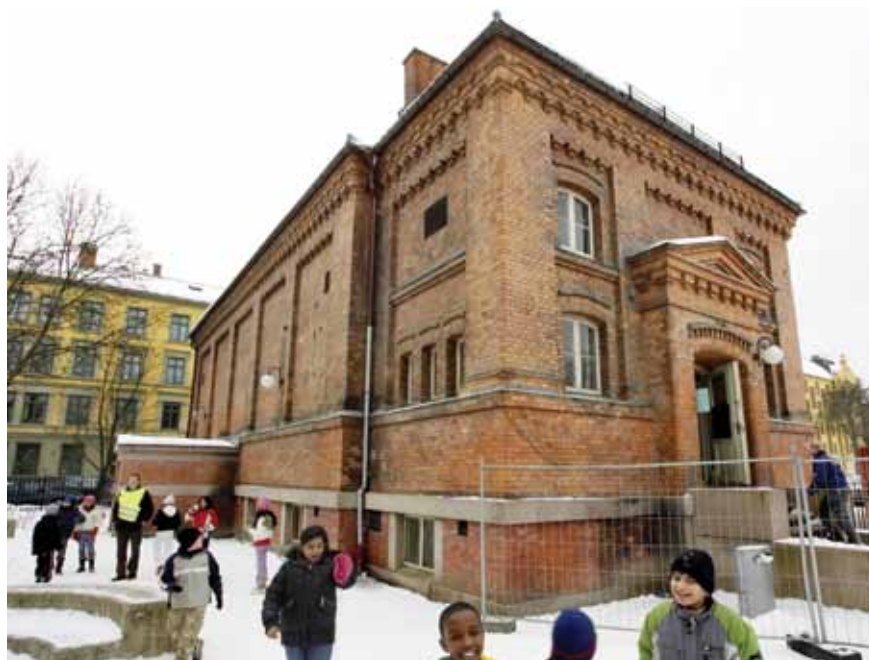
The Government's Stimulus Package resulted in several projects of school-renovation.
