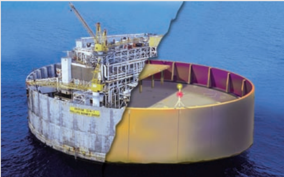
Figure 7.2 Illustration of the Ekofisk Tank before and after removal of the topsides
