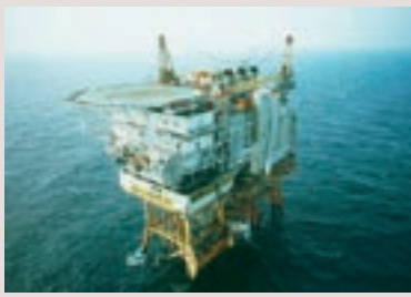
Figure 7.1 Installation 37/4-A, where the substructure is scheduled to be removed in summer 2010 (Source: ConocoPhillips Norge)
