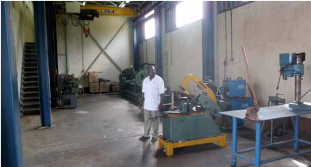
Hydropower plant workshop
