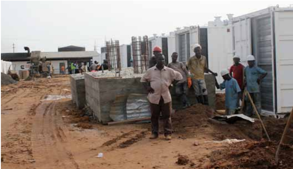
Emergency power supply to Monrovia
