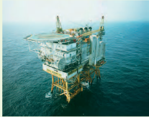
Figure 6.6 The pumping facility 37/4A whose substructure was removed during the summer (Source: ConocoPhillips)
