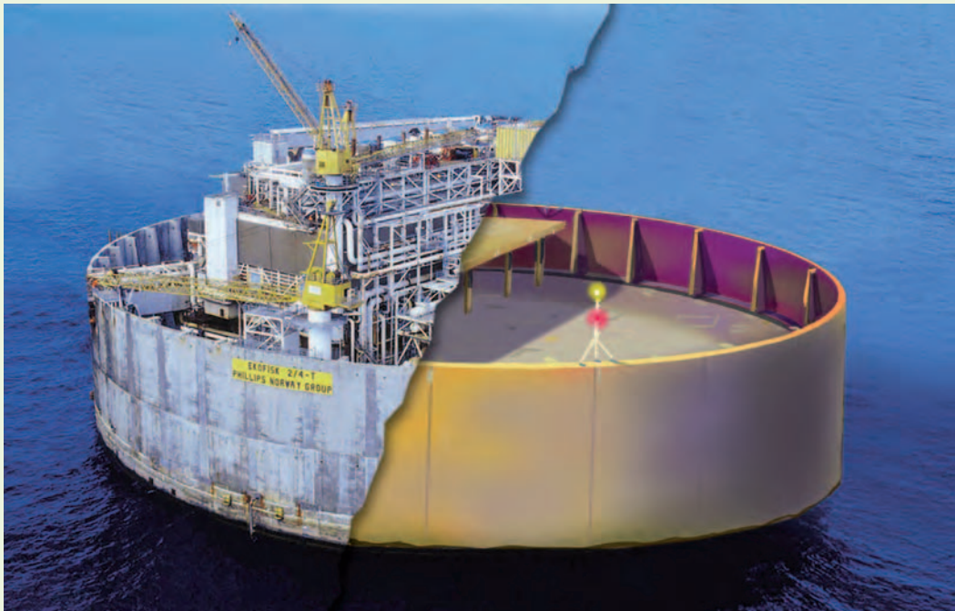
Figure 6.7 Illustration of the Ekofisk tank before and after removal of the topside (Source: ConocoPhillips)
