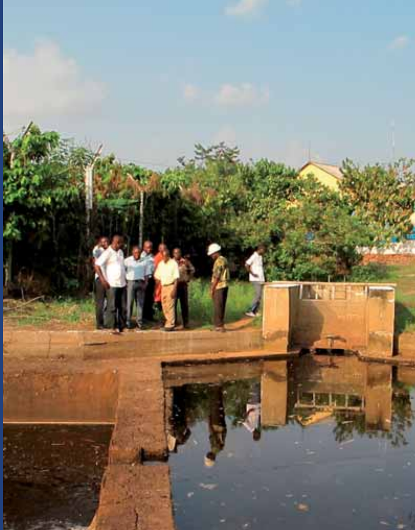
Inspection of a small irrigation dam in the Ashanti Region
