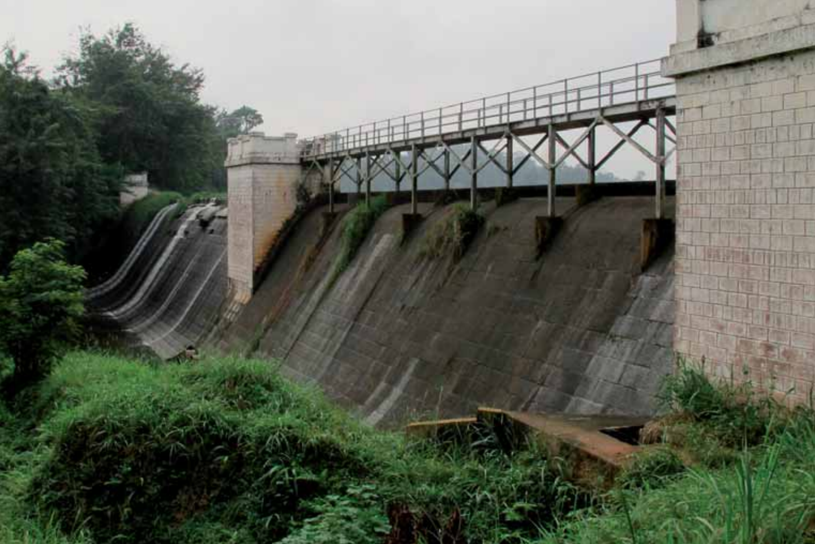
Dam in the Western Region of Ghana
