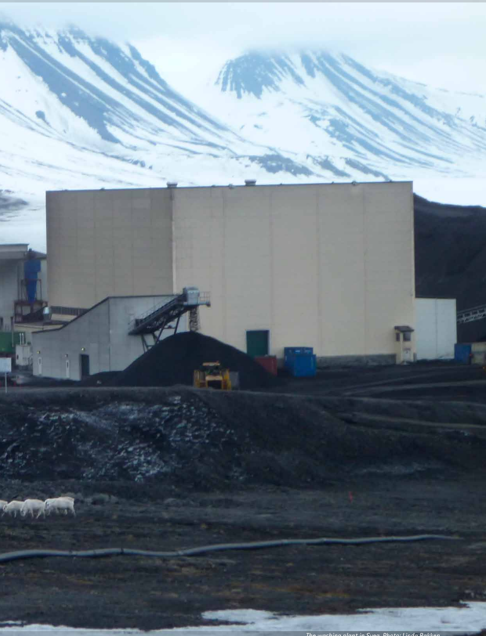
The washing plant in Svea. Photo: Linda Bakken
