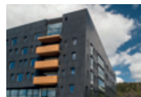
Builds Papirbredden 2 in Drammen
