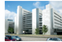
Renovates Fredrik Selmers vei 4 in Oslo
