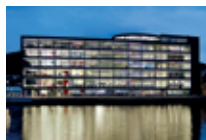
Builds Papirbredden in Drammen
