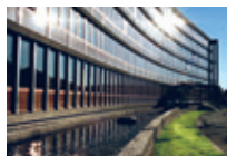
Renovates Middelthunsgate 29 in Oslo
