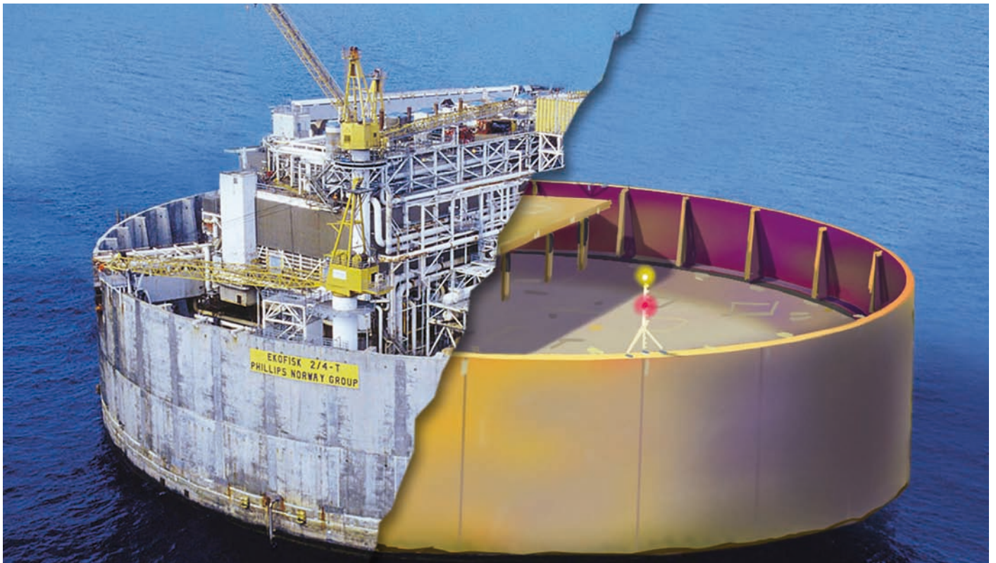
Figure 6.6 Illustration of the Ekofisk tank before and after removal of the topside (Source: ConocoPhillips)
