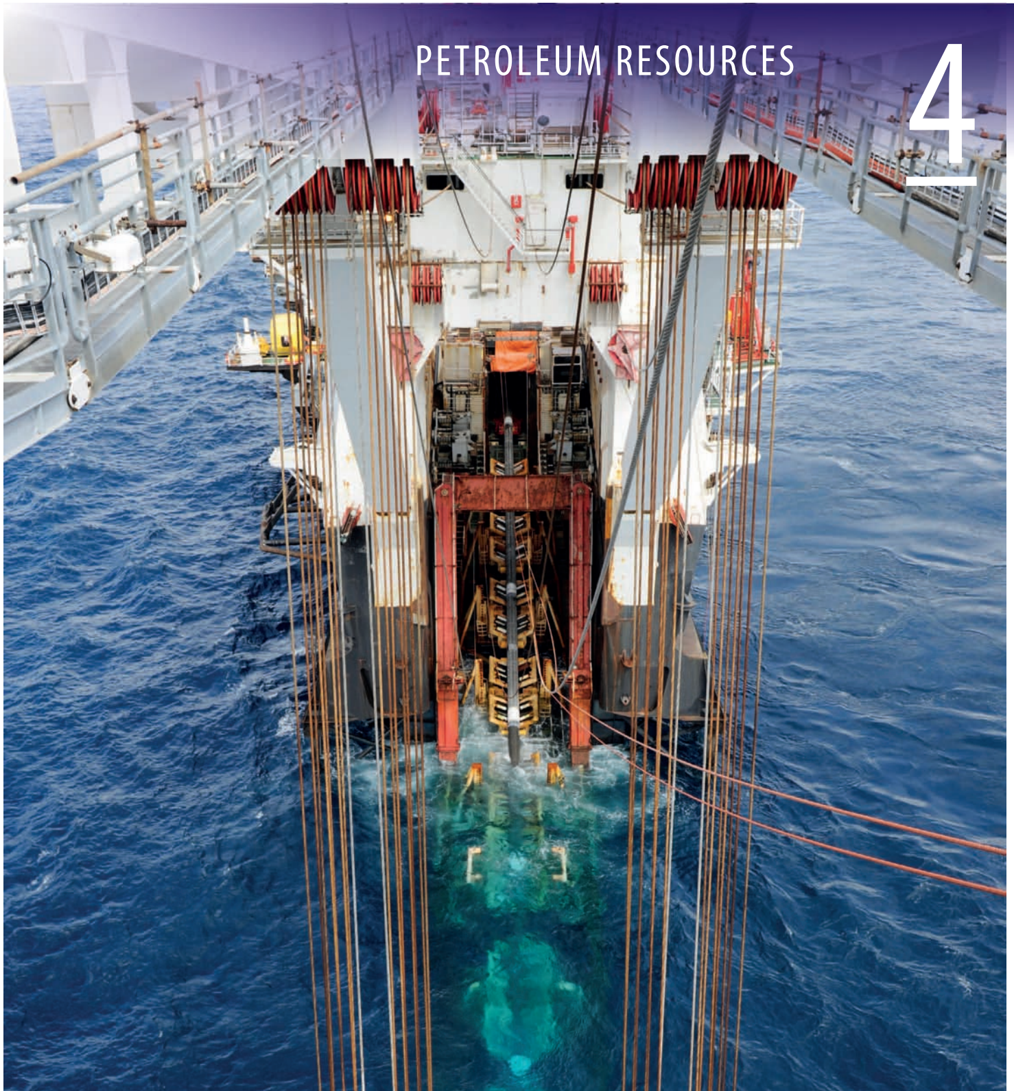
Pipelaying on the Ekofisk field, the first field on the Norwegian shelf. The field is expected to produce for another 40 years. (Photo: Kjetil Alsvik, ConocoPhillips)
