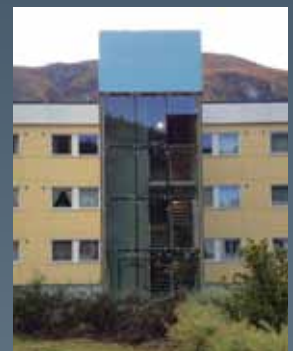
New lift shaft. Photo: Greta Steinheim, ABBL
