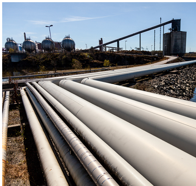
Johan Sverdrup pipeline installation at Mongstad, Norway
