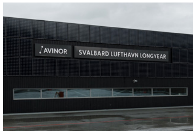
Solar panel array at Svalbard Airport.
