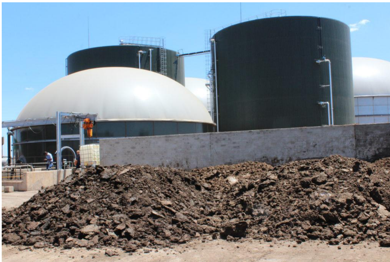
Bio2Watt in South Africa produces electricity from organic waste.
