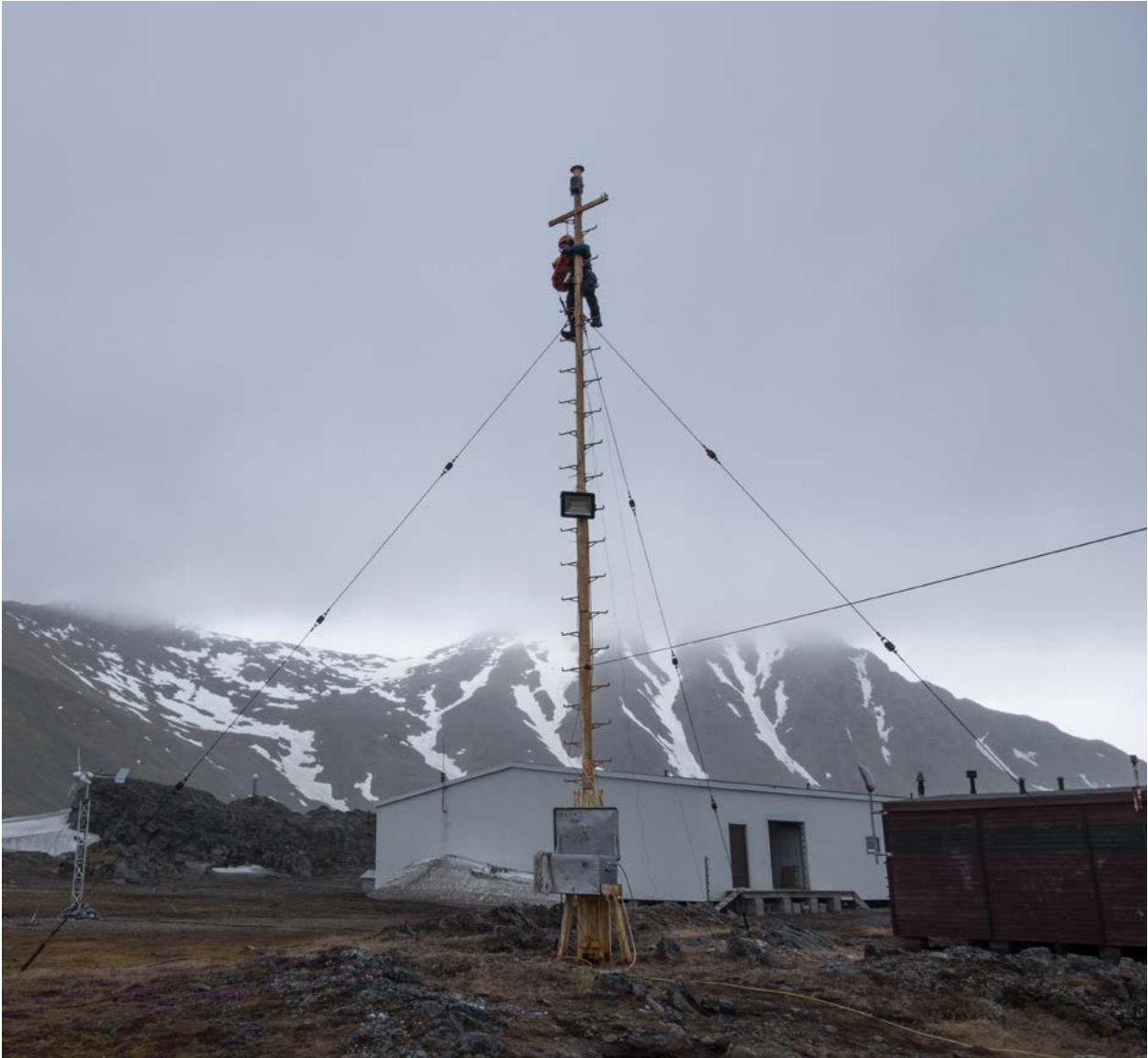
June 2020: Fixing a radar antenna at the Polish Polar Station in Hornsund. Photo: Mikko Syrjäsuo/UNIS.
