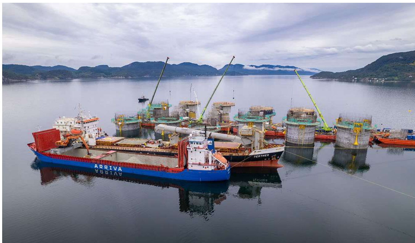
Slipforming at Dommersnes in July 2021, of substructures for Hywind Tampen floating offshore wind farm.
