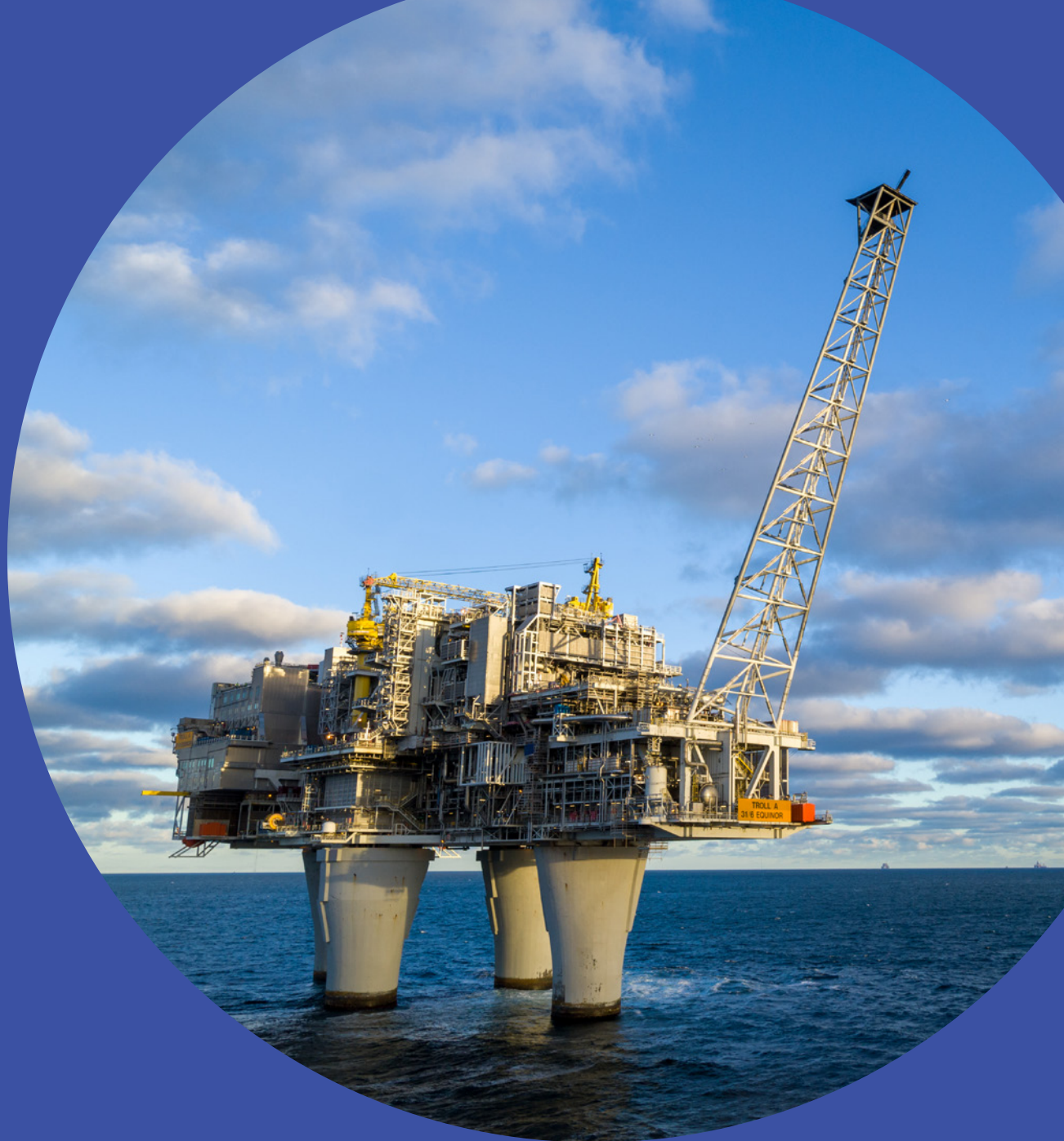
Troll A. Photo: Øyvind Gravås and Even Kleppa / Equinor
