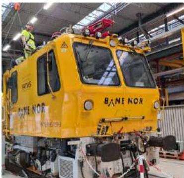
Raymond Lysaker fitting a roof antenna as part of the ERTMS project
