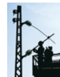
Installation of catenary
