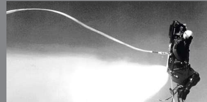
SEAT EJECTION BY ROCKET AND CATAPULTS FROM NAMMO PHOTO: NAMMO ARCHIVE
