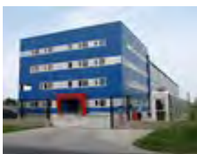
Romanian technology Heating
