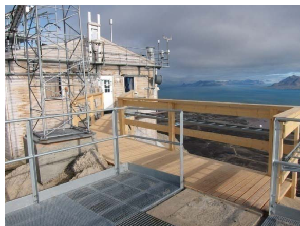
The new platform at Zeppelin Station
