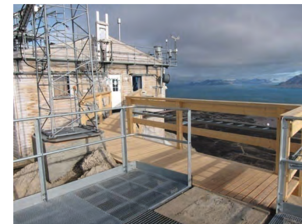
The new platform at Zeppelin Station
