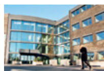
Rehabiliterer Prof. Olav Hanssens vei Stavanger
