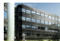
Rehabiliterer Powerhouse, Kjørbo
