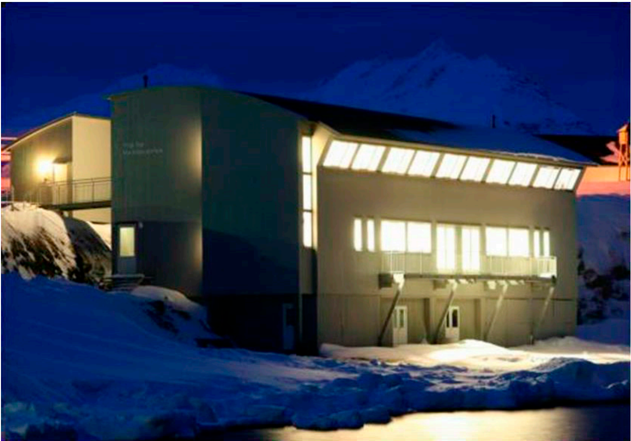
Kings Bay Marinlaboratorium.
