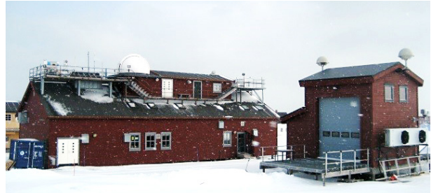
The new AWIPEV buildings, photo: Ole Øiseth
